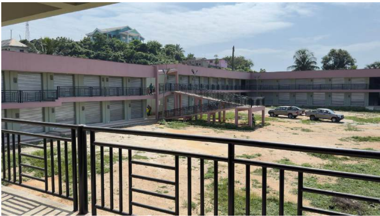
Construction of 60 Lockable Stores at Anomabo
