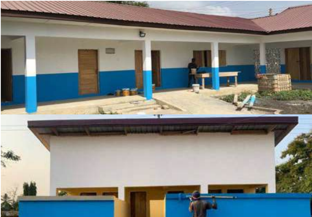
6 Classroom block with Toilet Facility at Oda
