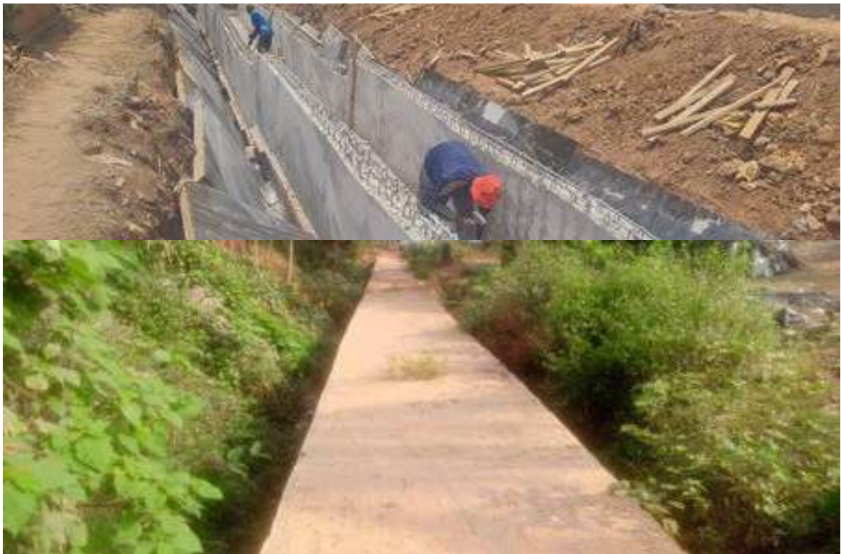
Storm Drain Work at Bohyen Kumasi
